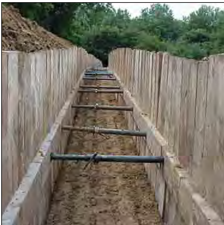
Plate 3.3 Timber shuttering to protect trench (if required)
