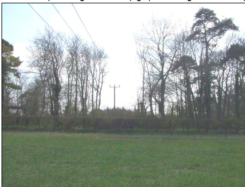
Plate 6.1 Carman’s Belt woodland (route aligned to west (right) of existing overhead line)
