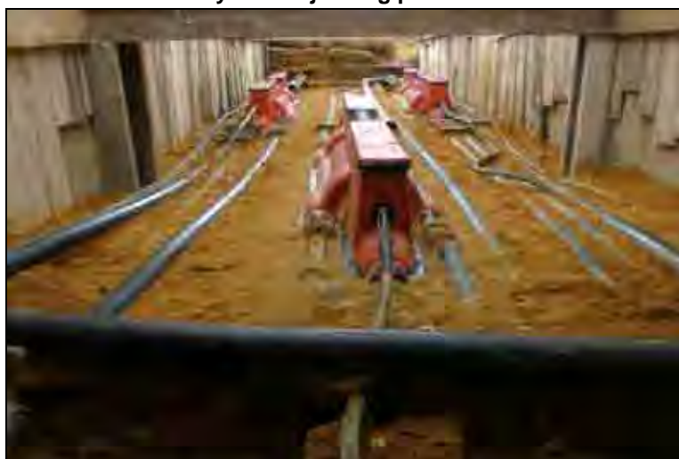
Plate 3.4 Partially buried jointing pit
